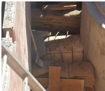
Figure 1 Formwork of Cast in Place Connection
