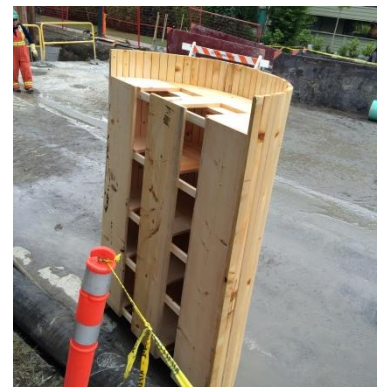
Figure 2 Cast in Place Channel Form Connection
