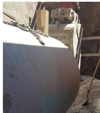
Figure 4 Excavator Driven Pipe
