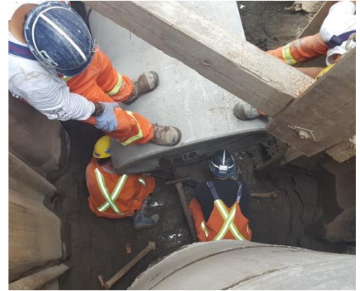
Figure 3 900mm RCP Being Jacked Into A Lok
